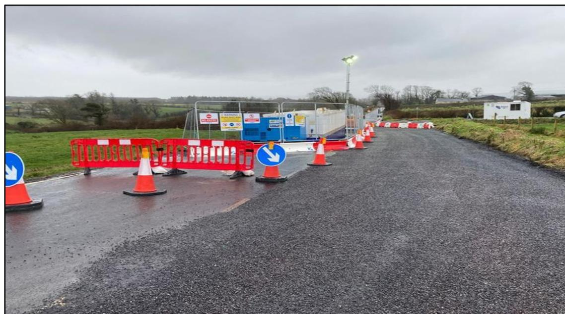
**Figure 2.7: Kilpaddoge-Knockanure 220 kV UGC project: Operational joint bay location comprising temporary welfare facilities, generator (blue cabinet), and jointing bay (white container over). A passing bay allows traffic flow around the joint bay – note natural revegetation of the edge of the passing bay**
