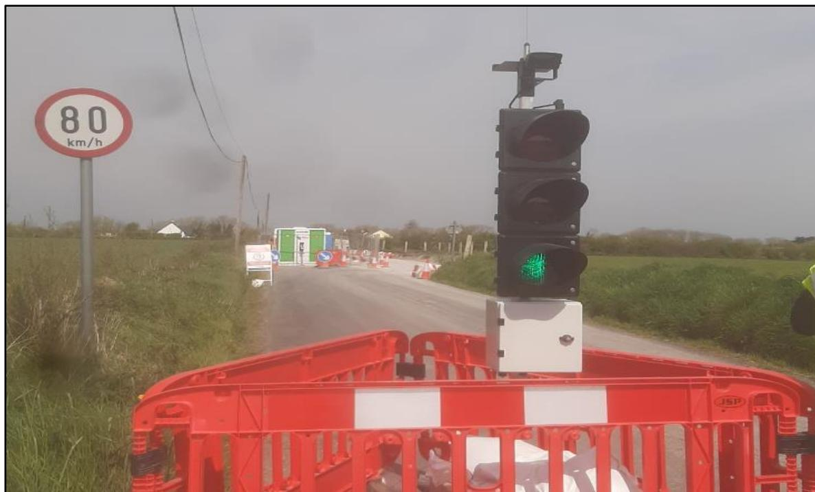
**Figure 2.6: Kilpaddoge-Knockanure 220 kV UGC project: Sensor controlled traffic management at operational joint bay and passing bay location**
