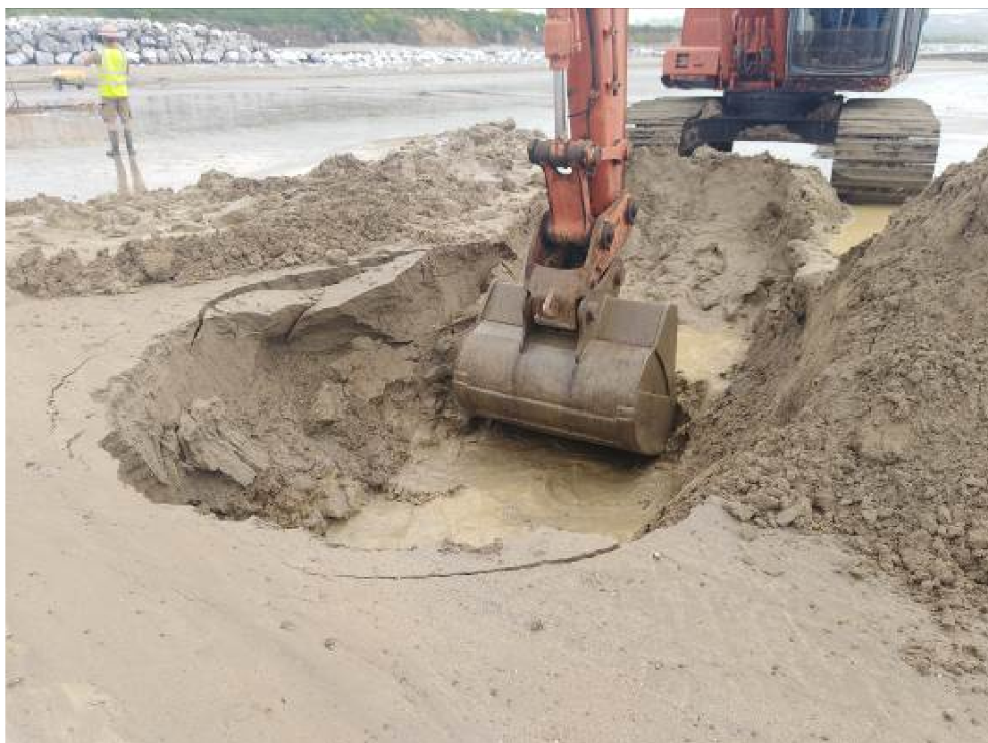
PLATE 4: BW2-TP2 during excavation, facing east
