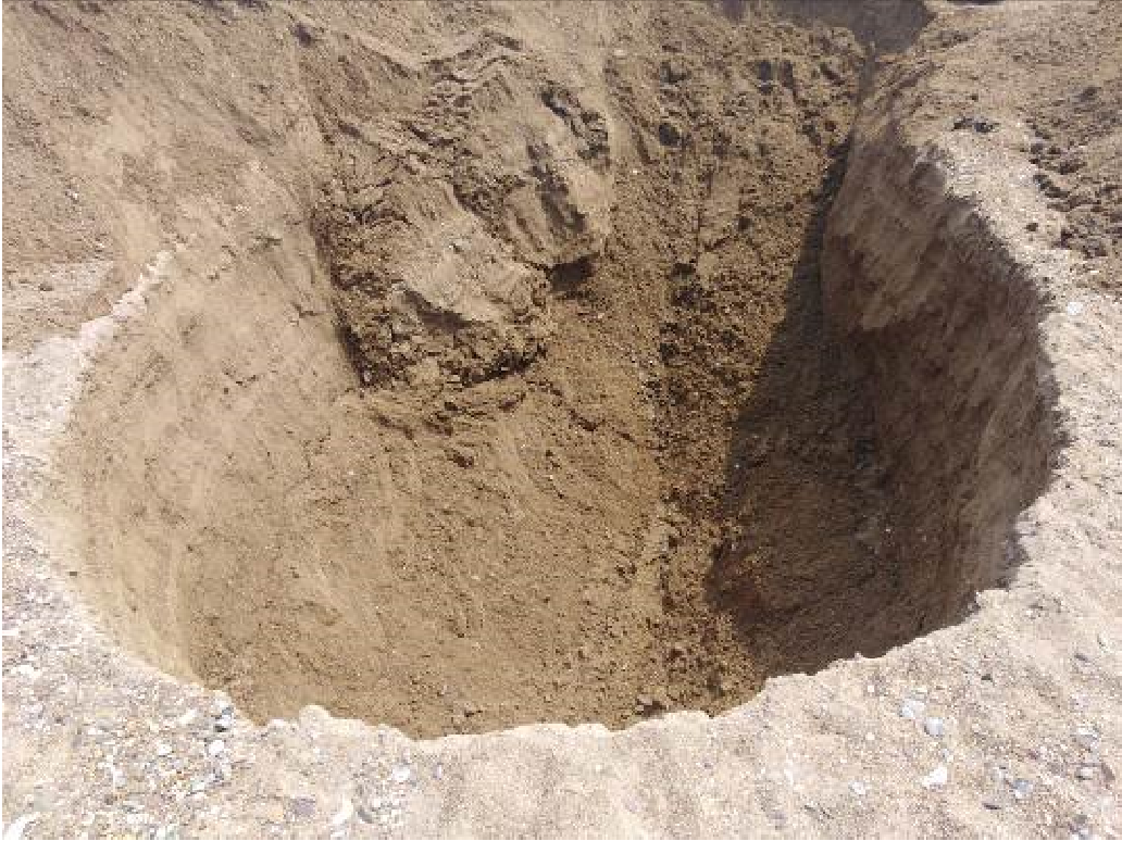
PLATE 9: CL-TP1 during excavation, facing southeast
