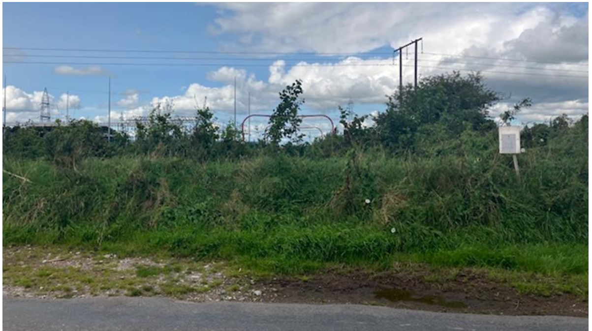
Photo 2: view to existing ditch at southern boundary of the Approved Cable Sealing End compound site at the location of the proposed vehicular access. This will require to be removed in any case to facilitate the laying of the Approved underground cables into the compound.
